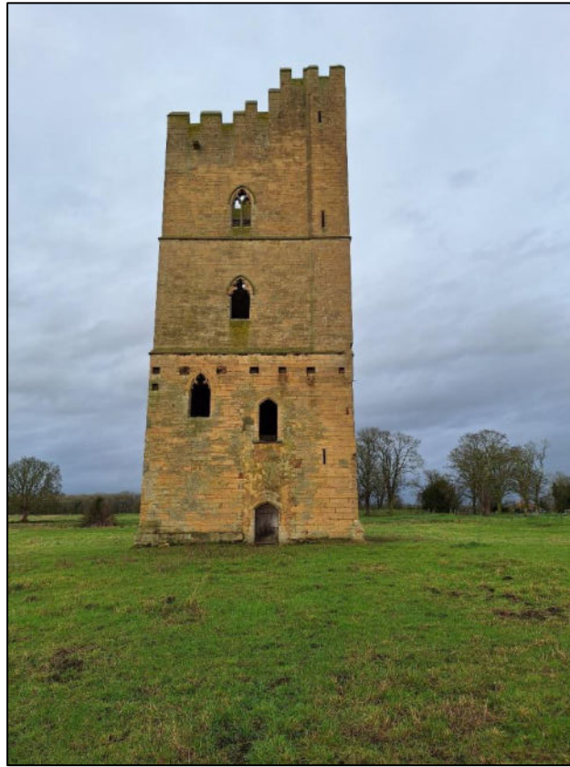
Plate 23: South elevation of Kyme Tower showing the bae slots for the ground and first floor where the earlier manor house was abutted onto the tower, the ground and first floor doorways are viewed.
